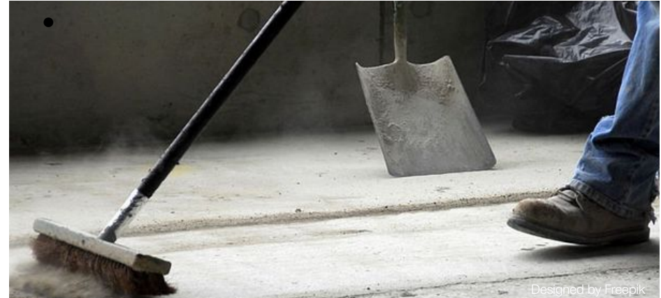
Image 22: Cleaning the laying area that will receive the ceramic coating.
