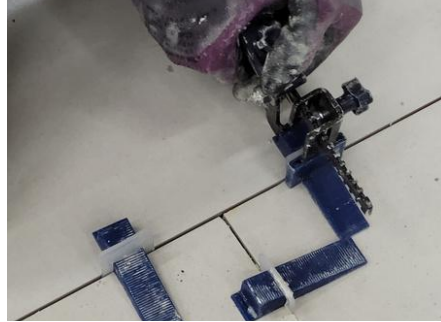
Image 36: Tighten with locking pliers.
