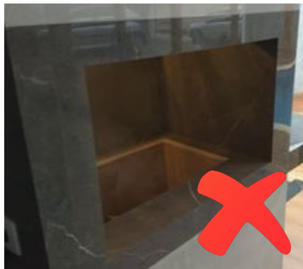
Image 10: The laying of a coating on the inside of the barbecue made of porcelain is not recommended, it should be refractory brick.
