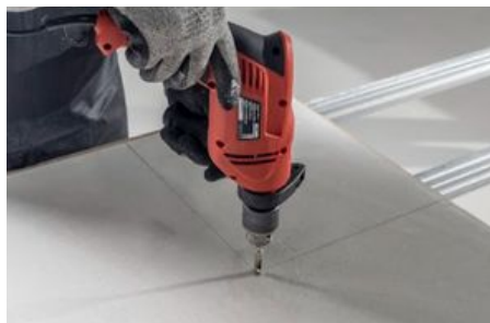
Image 85: Finish opening the four holes with the marble saw.
