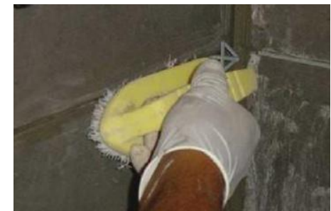
Image 34: Use a brush to clean excess mortar from the joints.
