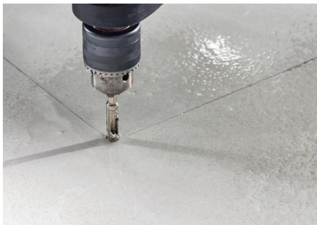
Image 80: Holes drilled at each 90° intersection.
