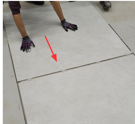
Image 30: Execution of dragging on the piece.
