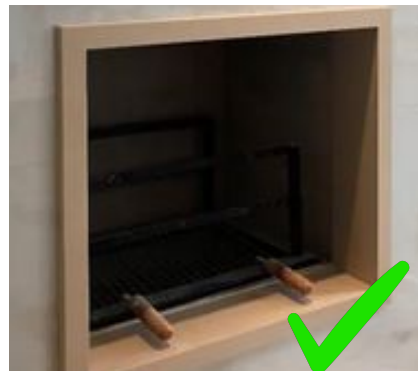
Image 11: It is recommended to use ceramic coating on the entrance and frame of the barbecue.
