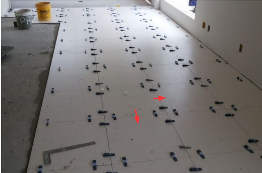
Image 42: Wedges in the same row must be inserted in the same direction.
