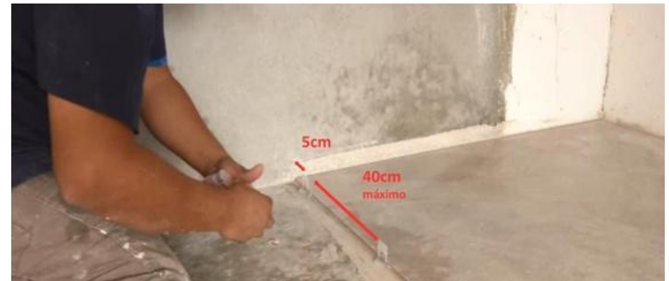
Image 41: Clip spacing patterns in the piece.
