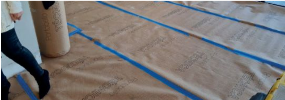
Image 46: Applied floor protector
