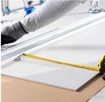
Image 70: Marking the rail fitting.
