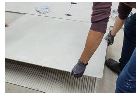
Image 33: Execution of dragging on the piece.
