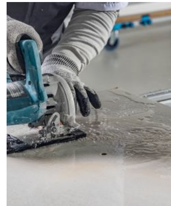
Image 87: Finish the cut opening at the hole with the marble saw.
