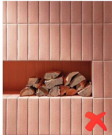
Image 16: It is not recommended to apply ceramic coating to the inside of traditional barbecues and wood-burning fireplaces.
