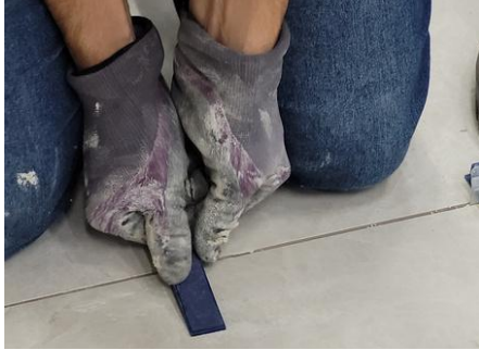
Image 35: Insert the wedge into the clip manually.
