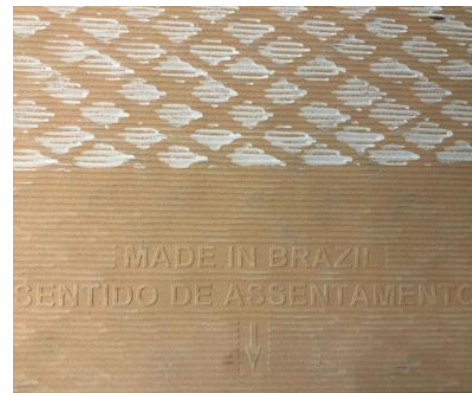
Image 23: Arrow in high relief on the reverse of the piece.
