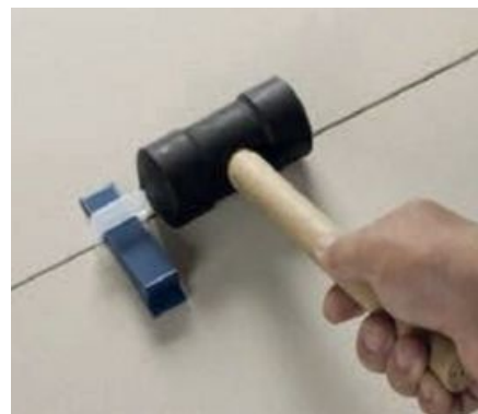
Image 44: Removal of clip and wedge.
