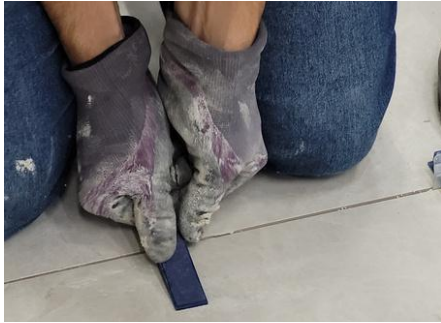
Image 35: Insert the wedge into the clip manually.
