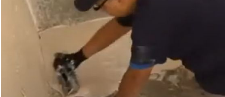
Image 25: Apply mortar to the laying area with the smooth side of the trowel.
