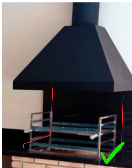
Image 15: Ceramic coating on grill barbecue with joint indications.
