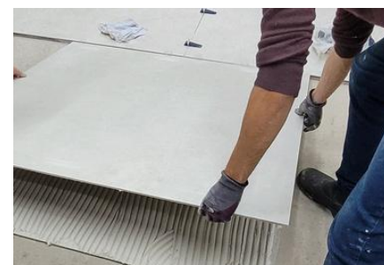
Image 33: Execution of dragging on the piece.
