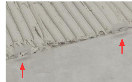
Image 32: Leveling spacer
