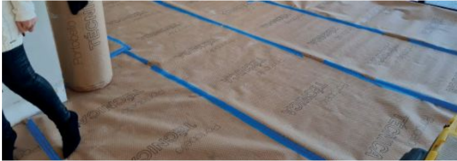
Image 46: Applied floor protector
