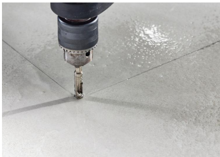
Image 80: Holes drilled at each 90° intersection.
