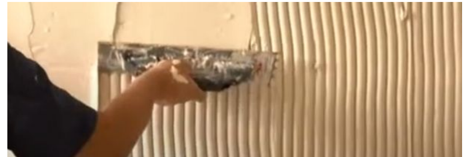
Image 28: Opening of mortar grooves in the ceramic coating with the toothed side of the trowel.
