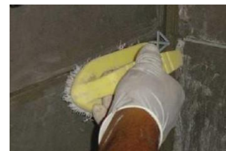
Image 34: Use a brush to clean excess mortar from the joints.
