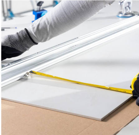
Image 70: Marking the rail fitting.
