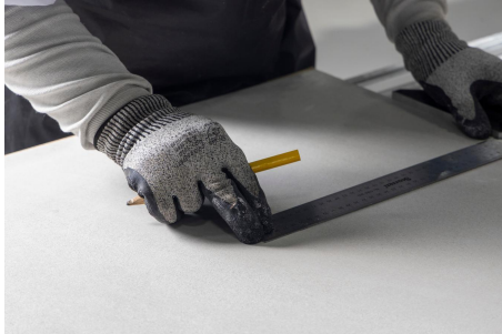
Image 52: Cut marking at the ends.
