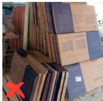
Image 04: Improper stacking.
