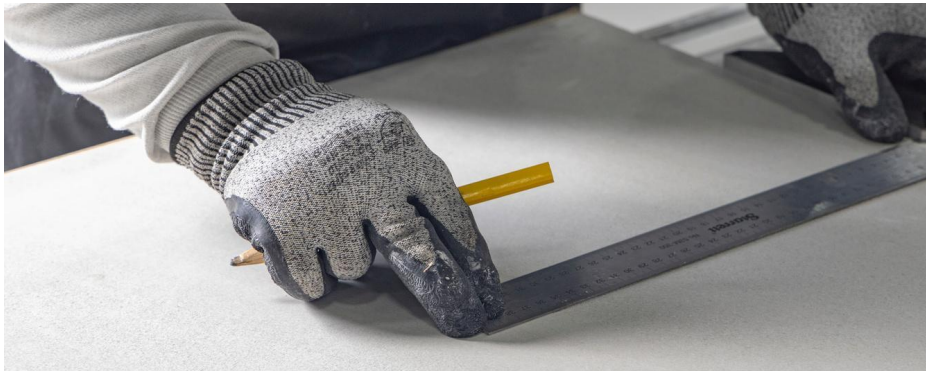
Image 84: Draw the cut to be made on the piece.
