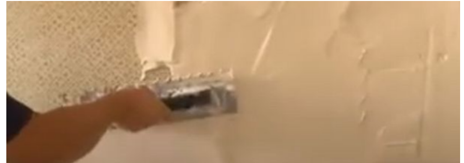
Image 27: Application of mortar to the ceramic coating with the smooth side of the trowel.
