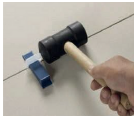
Image 44: Removal of clip and wedge.
