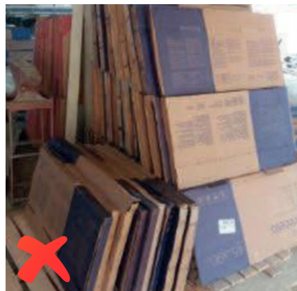
Image 04: Improper stacking.
