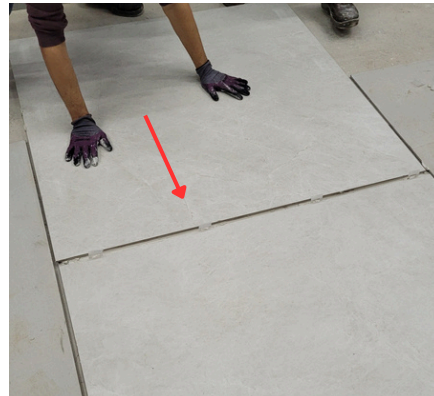
Image 30: Execution of dragging on the piece.
