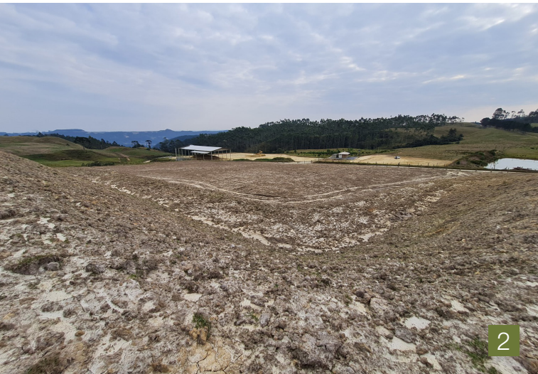
(1) Beginning of environmental recovery of Leoberto Leal/SC/Slope and Bench (2) Recovery after the return of the fertile soil layer (3) Recovery after sowing grasses: the original vocation of the land was livestock farming and also agriculture
